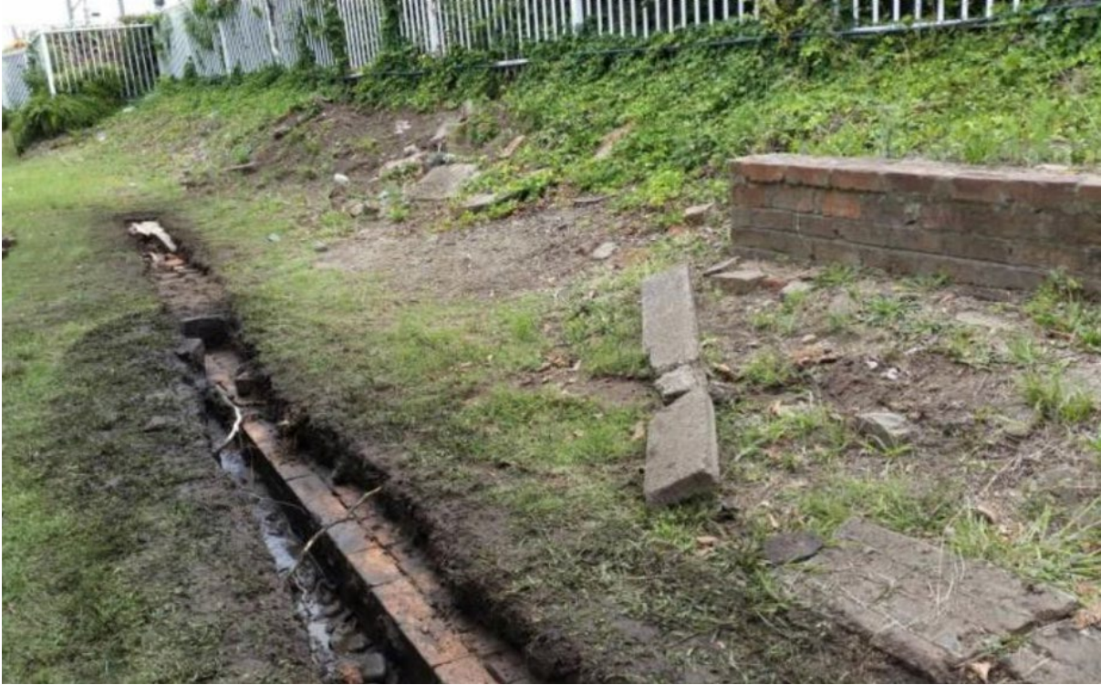
Figure 6: Platform at Hamilton Station classified as a 'work' by the project archaeologist, Wickham Transport Interchange project, 2015
