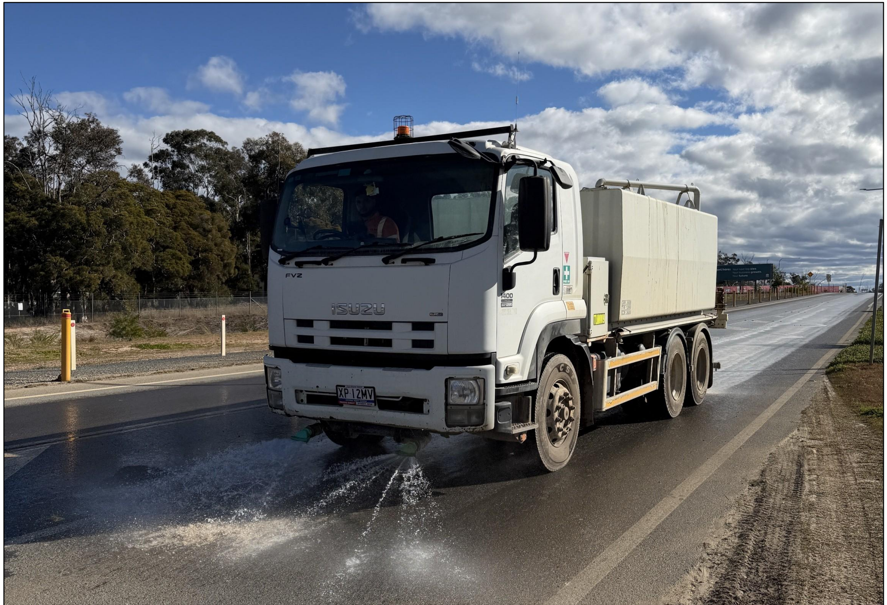
PHOTO 7 POLYMER APPLICATION WORKS CAPTURED ON 10.03.2026
