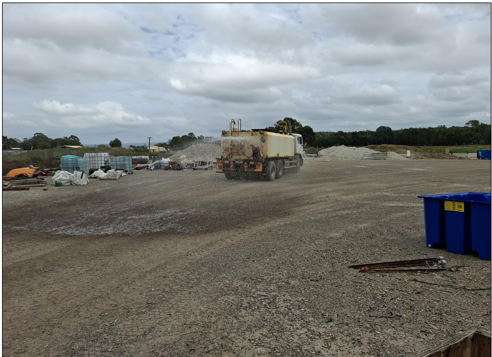
PHOTO 6 DUST SUPPRESSION WORKS CAPTURED ON 10.03.2026
