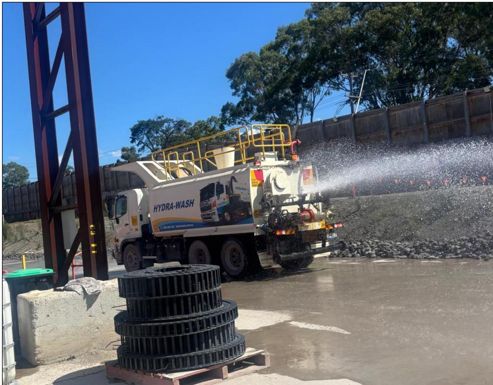
PHOTO 9 DUST SUPPRESSION WORKS CAPTURED ON 22.10.2025
