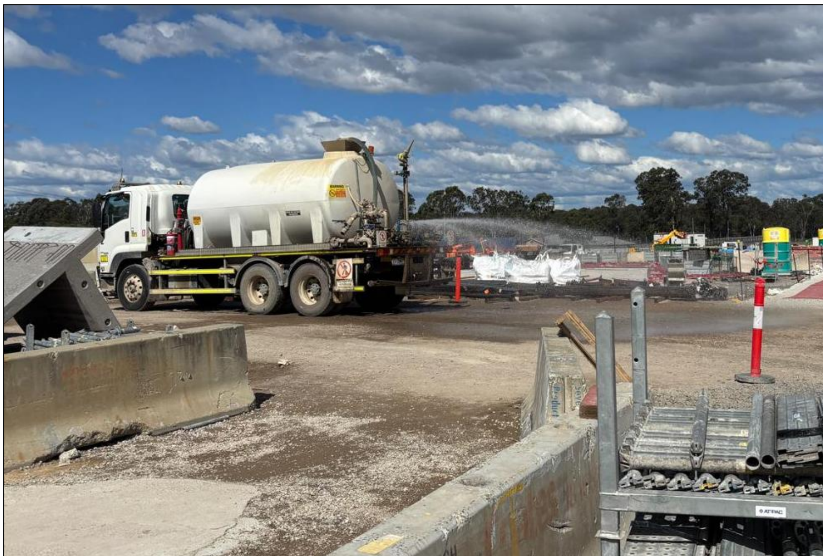
PHOTO 10 DUST SUPPRESSION WORKS CAPTURED ON 29.08.2025
