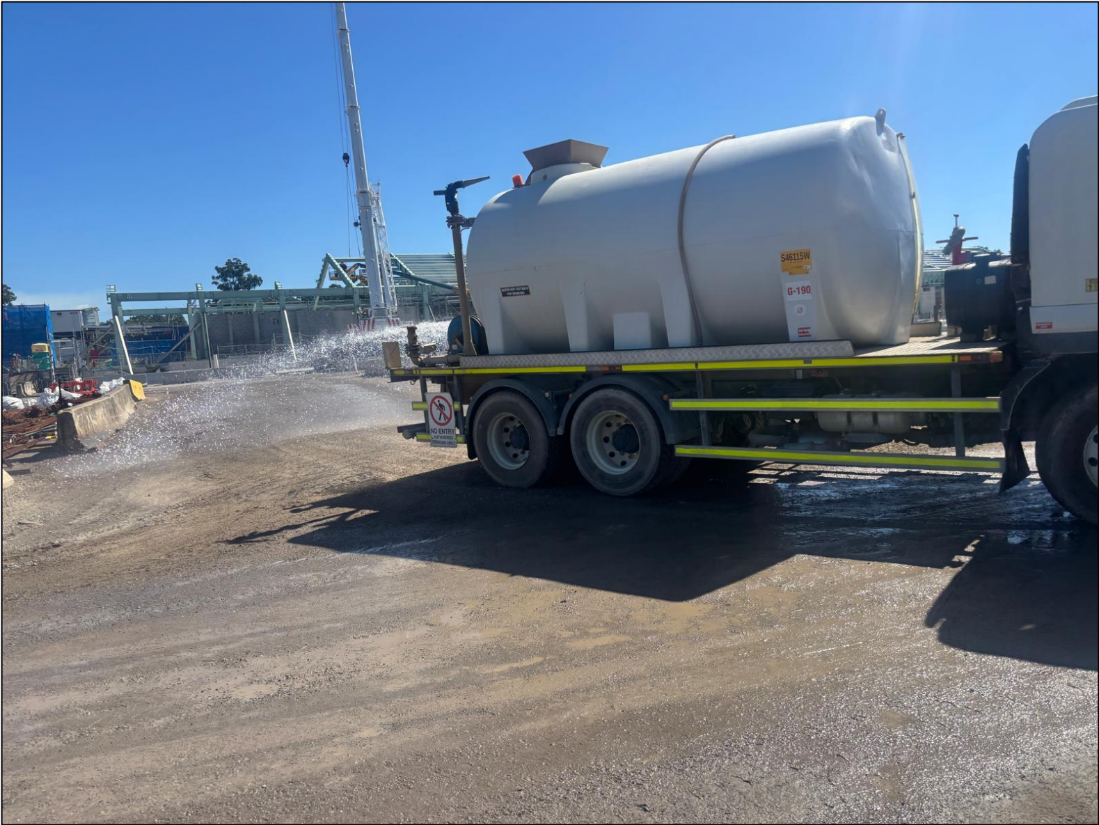
PHOTO 1 DUST SUPPRESSION WORKS CAPTURED ON 01.04.2026
