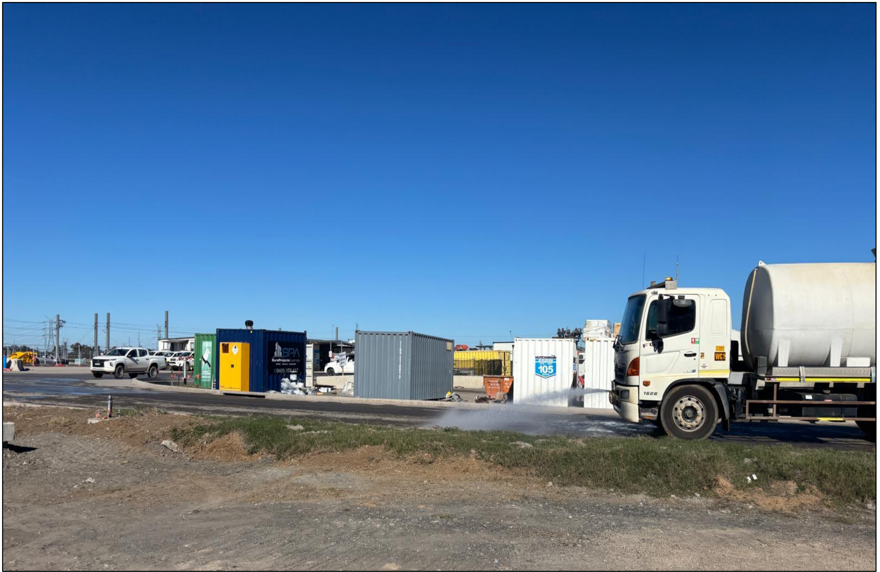
PHOTO 3 DUST SUPPRESSION WORKS CAPTURED ON 24.07.2026
