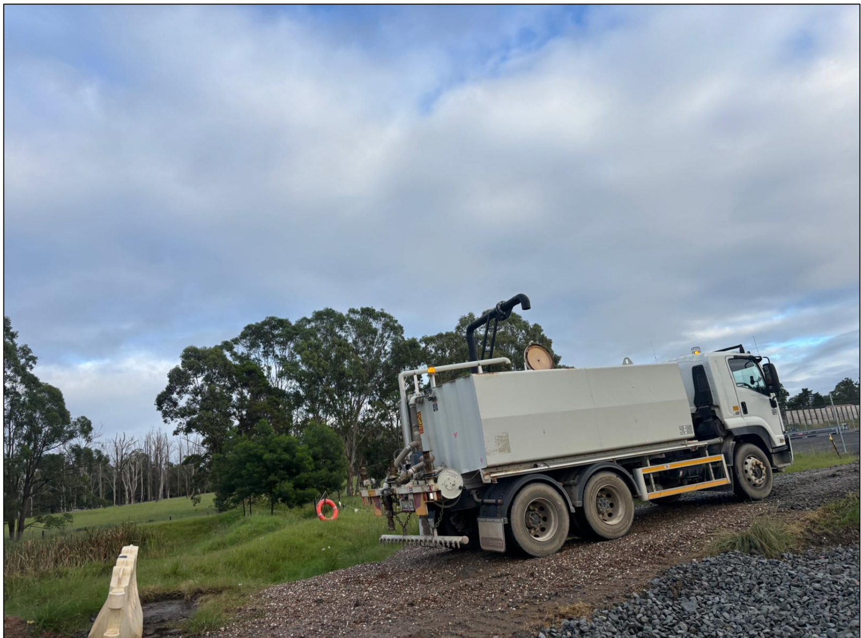
PHOTO 8 WATERCART FILLING FOR DUST SUPPRESSION CAPTURED ON 02.03.2026
