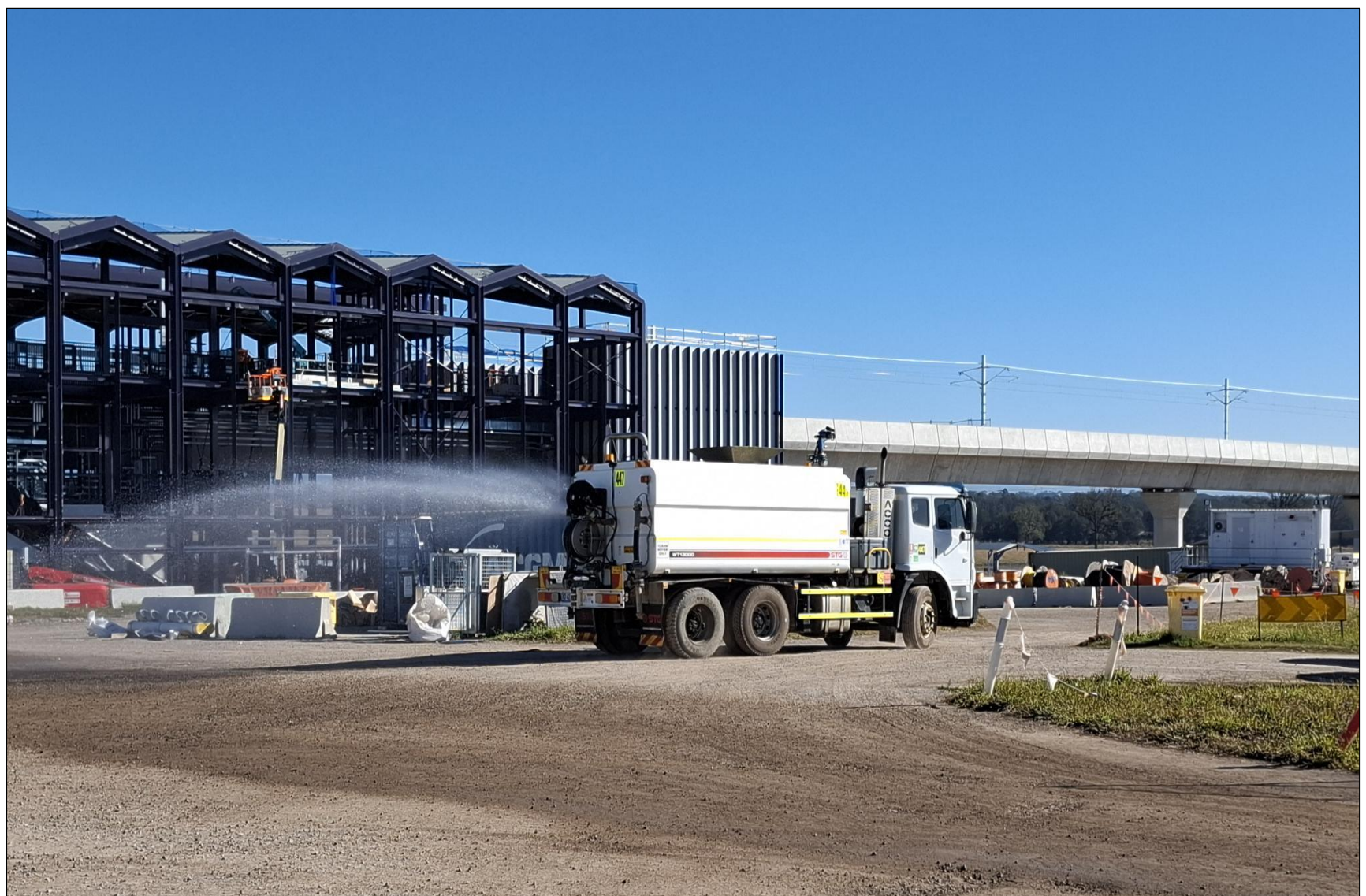
PHOTO 4 DUST SUPPRESSION WORKS CAPTURED ON 03.02.2026
