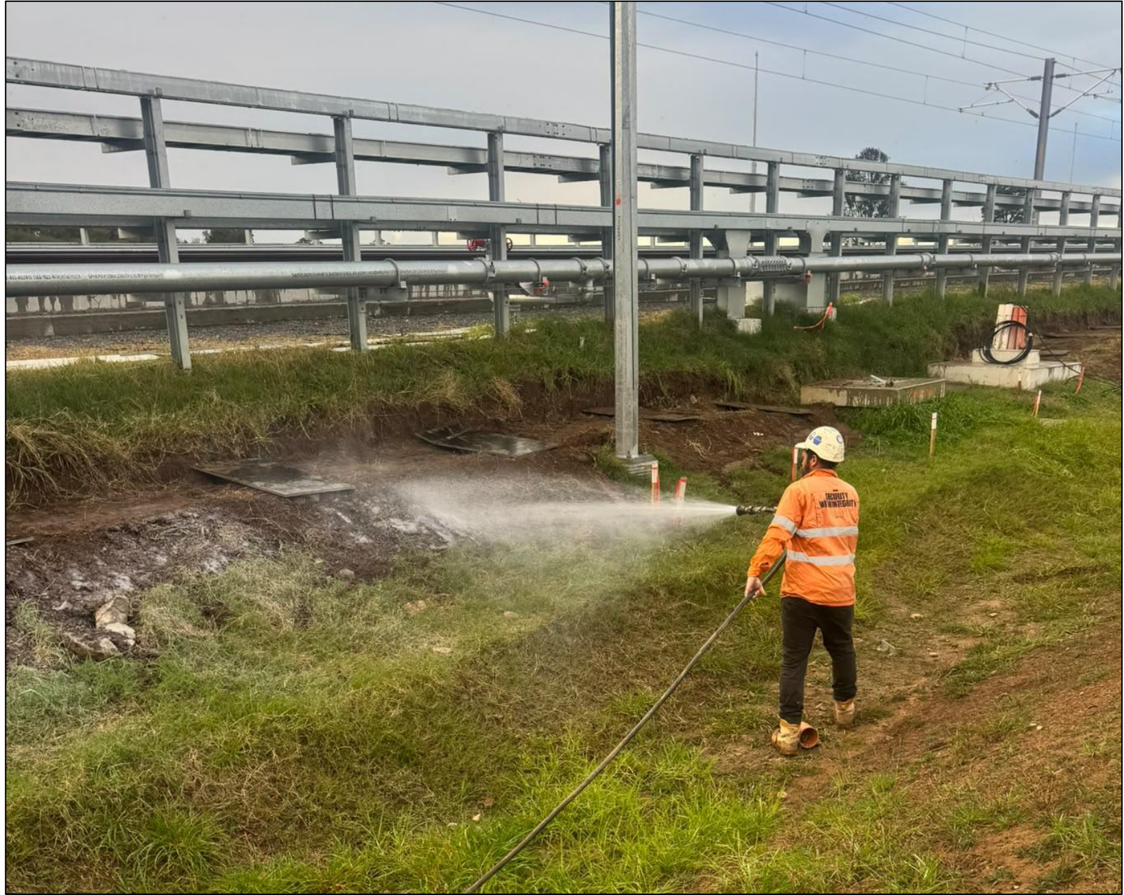
PHOTO 5 POLYMER APPLICATION WORKS CAPTURED ON 13.07.2026
