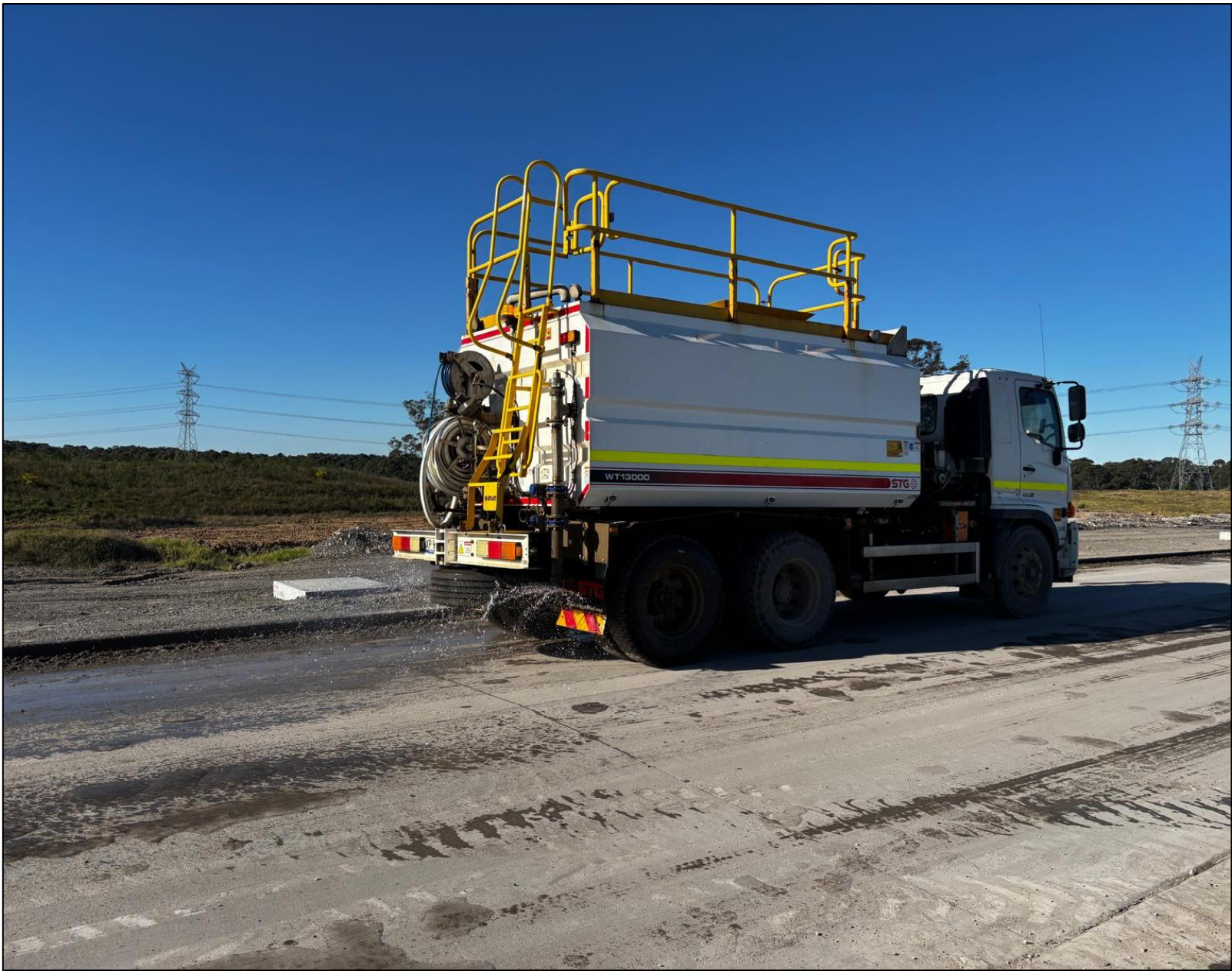
PHOTO 2 DUST SUPPRESSION WORKS CAPTURED ON 24.06.2026
